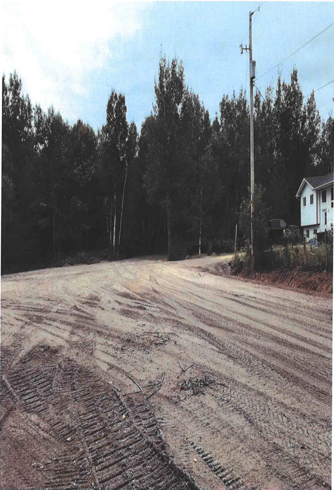
New Turn Around at Ground Hog Corner.
